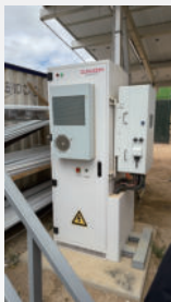
South Africa OASIS 60 & Deye 50kW/120 kWh Outdoor Battery Cabinet System
